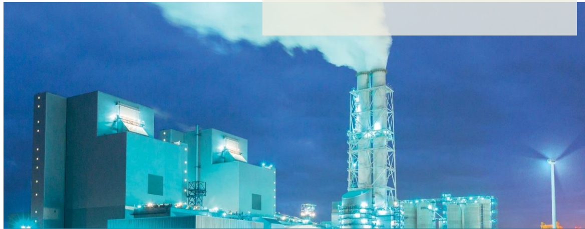
Client: RWE Technology GmbH - Period: 2008 - 2017
