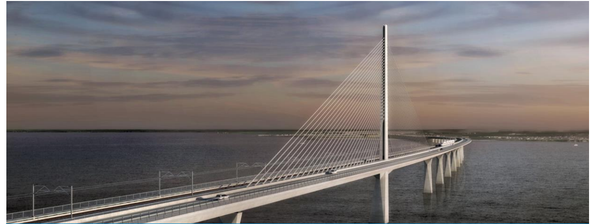
Client: SBJV Storstrøm Bridge Joint Venture - Period: 2018
